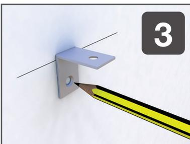
Offer your top brackets up to the lines and mark the holes before drilling and fixing as you did in Step 1. Make sure you position the bracket correctly - the inside of the top leg should be on the line.
