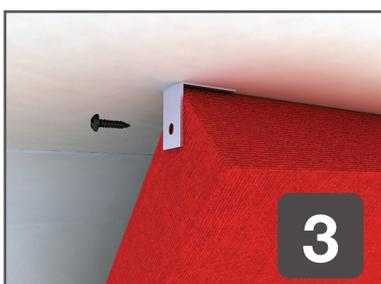
As per Section A and B, mark and fit 2 L Brackets at the far end of the trap and fix into the MDF edging of the trap with 4 'pan head' wood screws.
